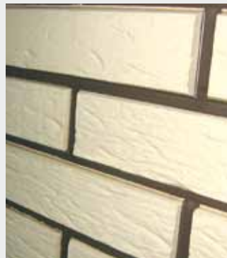
Sharp-edge paint application without a stencil
