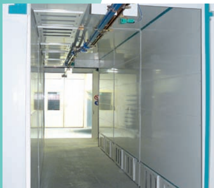
Conveyors and drying systems
